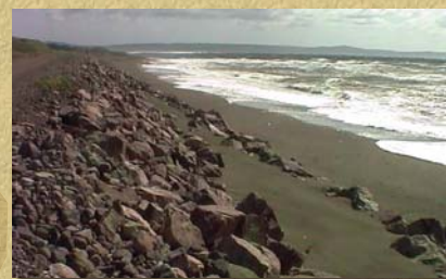
Enrochements. Photo DAF.
